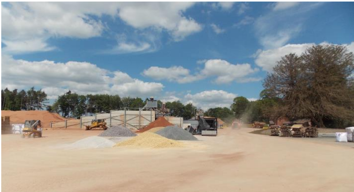
Figure 5 – Quarry plant site
